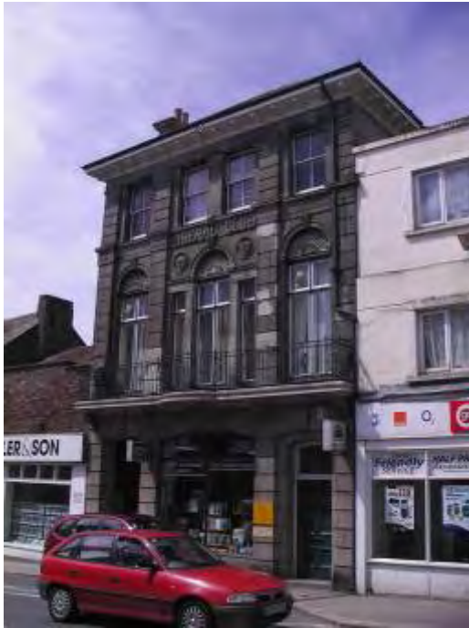
Rusticated granite ashlar blocks on the façade of a late nineteenth century shop on Barras Street
