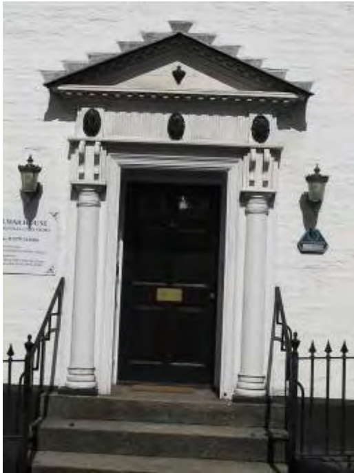
The doorcase to Kilmar House is designed in the classical style with pedimented doorway with engaged Tuscan columns to consoles; moulded architrave; entablature with paterae and dentilled cornice; fielded panelled reveals and 6-panel door
