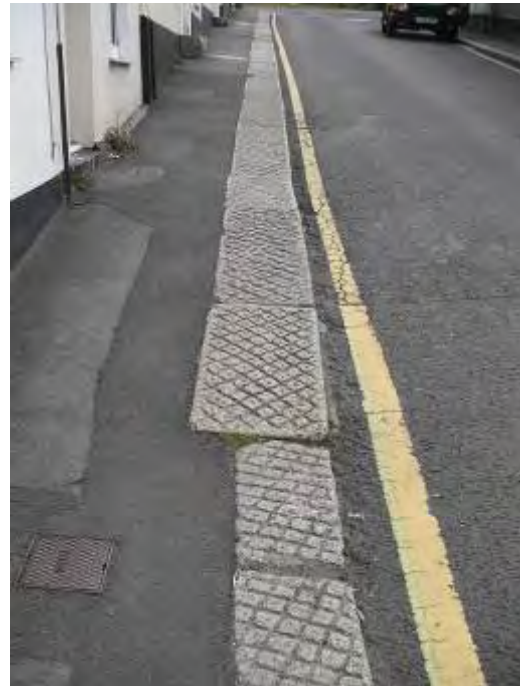
Wide granite kerbs with distinctive diamond pattern on Church Street North
